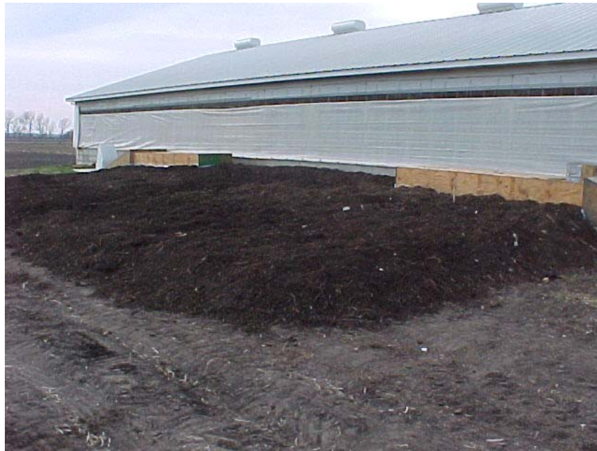
Figure 4. Biofilter built on a curtain-sided pig finishing barn (west half) with curtain closed
