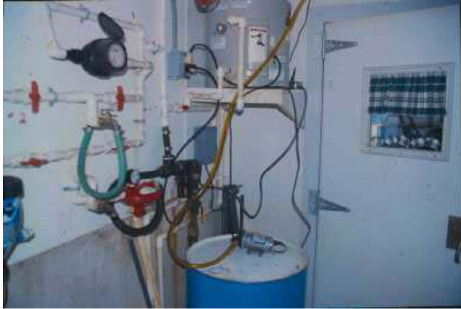
Figure 2. Injection oil pump and storage barrel plus plumbing for oil sprinkling system.
